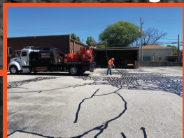
Crack Sealing
