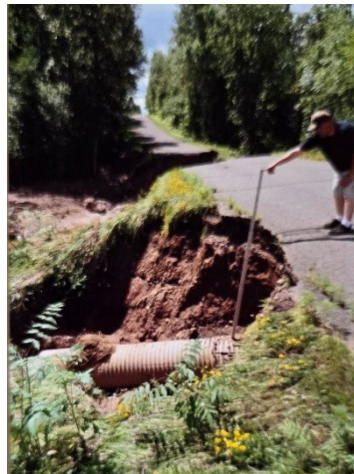
Culvert damage and washed out roads after the July 2016 storm. Photos courtesy of the Town of Marengo.
