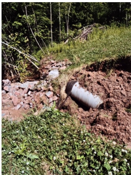
Culvert damage and washed out roads after the July 2016 storm. Photos courtesy of the Town of Marengo.
