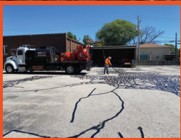
Crack Sealing
